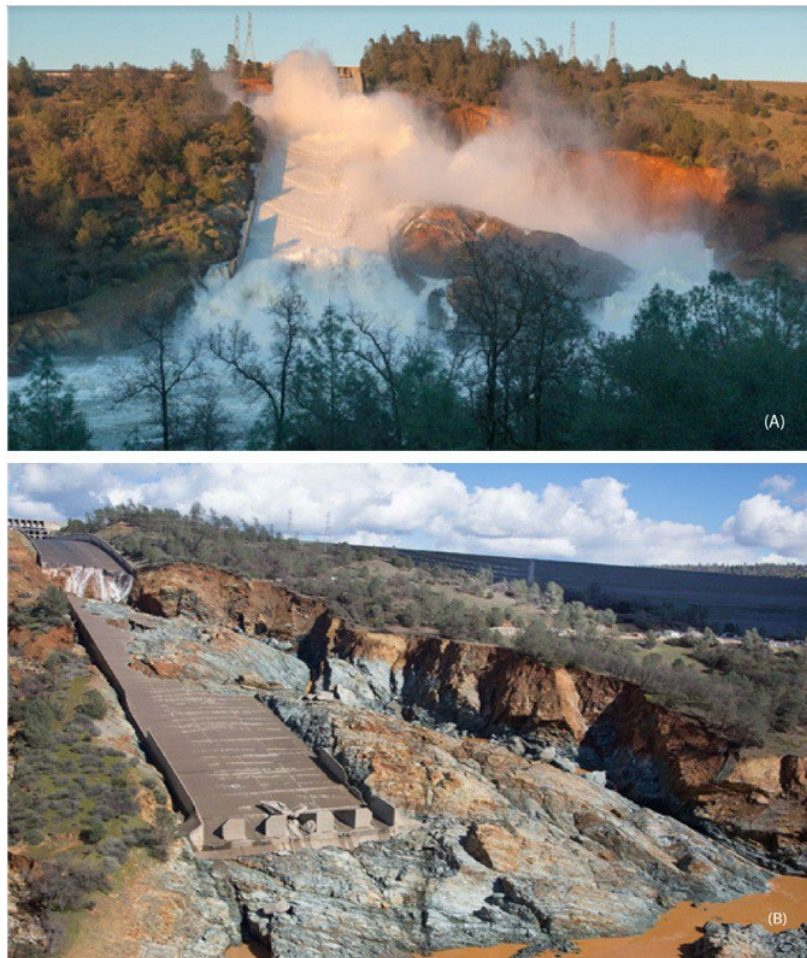
Figure 3. Views of the Main Spillway (A) during post-failure managed emergency discharge in February 2017, and (B) shortly after shutdown for emergency repairs in March 2017. Note the extreme erosional damage from flow channelization at the right (southeast) side of the image.
