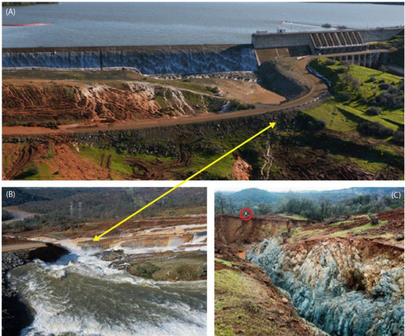
Figure 4. Views at the Emergency Spillway (A) during overtopping on February 11, (B) downstream view from the crest during peak flows, showing washout of the access road ( arrow indicates relative location), (C) post-flow, near the former access road, showing extent of downstream erosion and channelization (Photo by author; note the human inspector in the background (circled for scale)).
