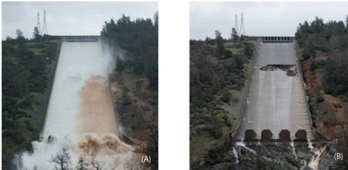
Figure 2. The Main Spillway at time of first damage (A), February 7. and (B) shortly after shutdown showing initial damage.
