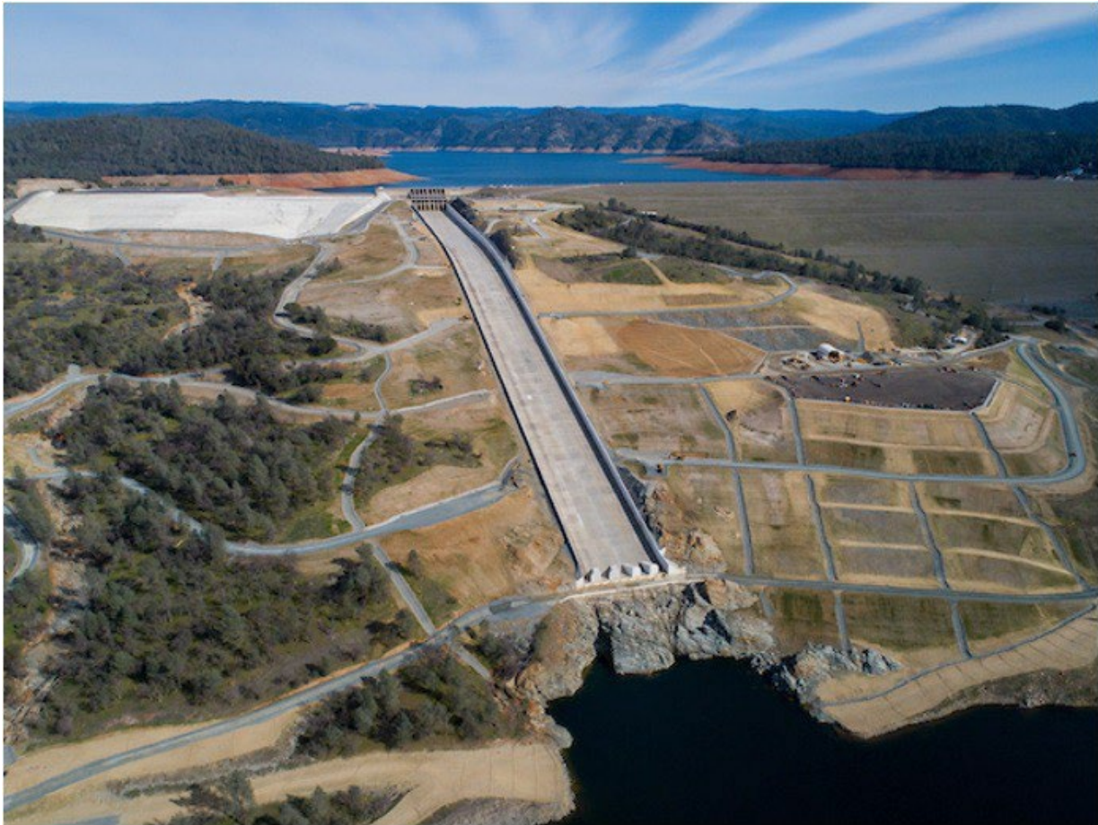
Figure 13. Oroville Dam Main Spillway and Emergency Spillway in 2020, after completion of reconstruction efforts.
