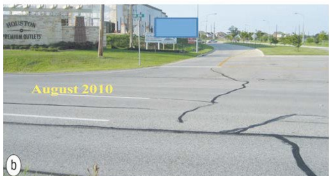
Figure 14. Recent pictures of Hockley fault at Highway 290 Frontage and Fairfield Falls Way roads: (a) taken in April 2010 and (b) taken in August 2010. Note the development of the tiny cracks in (a) into significant cracks in (b).
