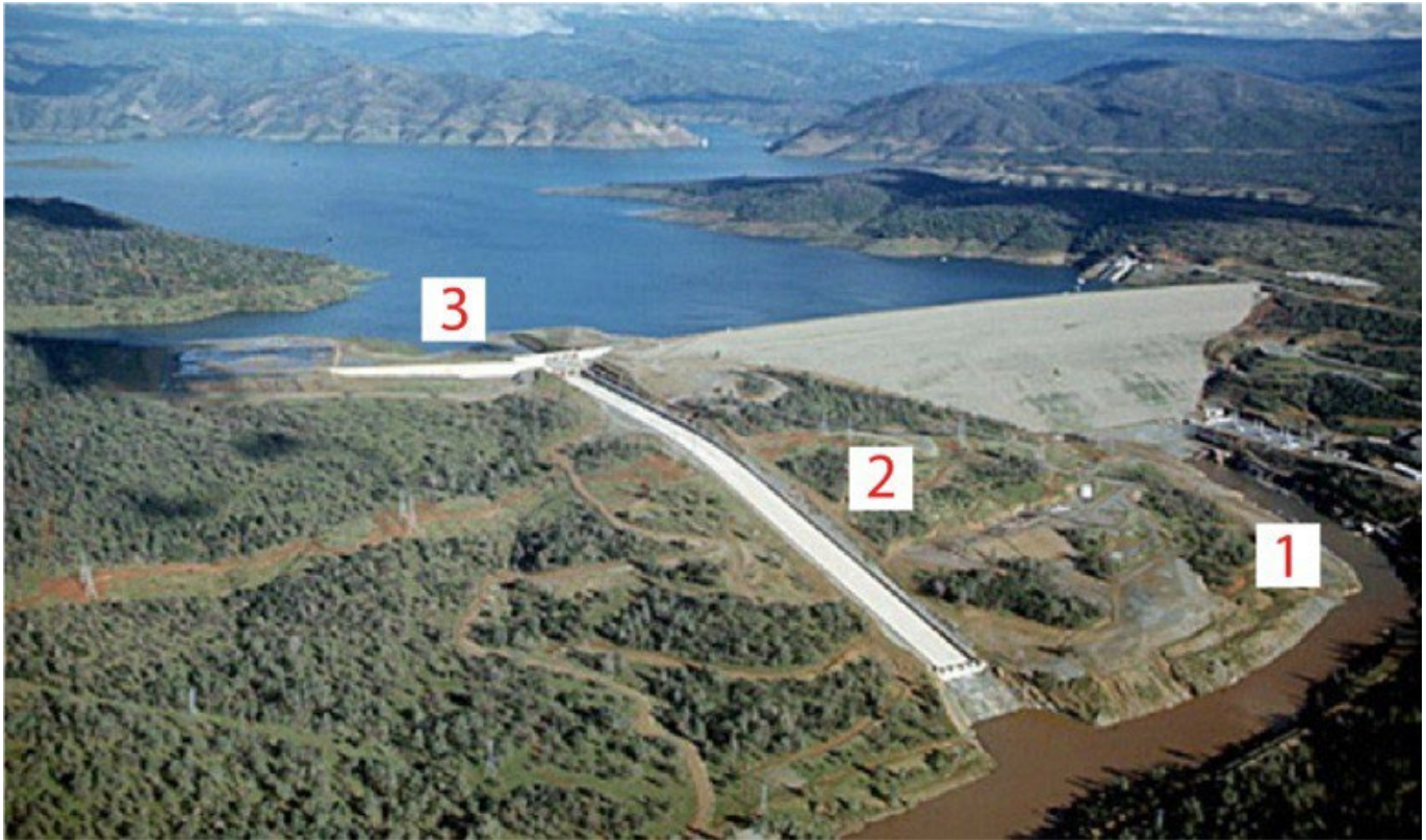
Figure 1. Lake Oroville Dam and Reservoir, circa 2015 (before spillway failure). Outflows from the reservoir are controlled from the three locations: 1) power plant, 2) Main Spillway, and 3) Emergency Spillway.
