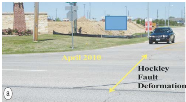
Figure 13. Photo showing the location of Fault B on the East-bound feeder road. Note that the fault is expressed as a discrete, linear rupture, which has been filled with asphalt. Resistivity and GPR data are collected along the yellow line.
