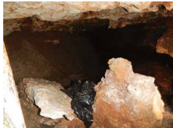
Figure 16: A picture showing the part of the cave which was encountered during the excavation.
