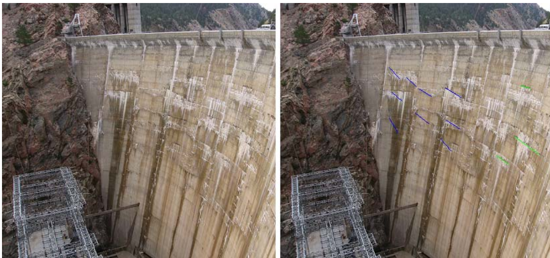
Figures 5.a and 5.b: Photographs taken during data collection of the downstream face of the dam, viewing the right abutment. 4.b highlights some obvious fractures, with steeper fractures highlighted in blue and horizontal fractures in green.
