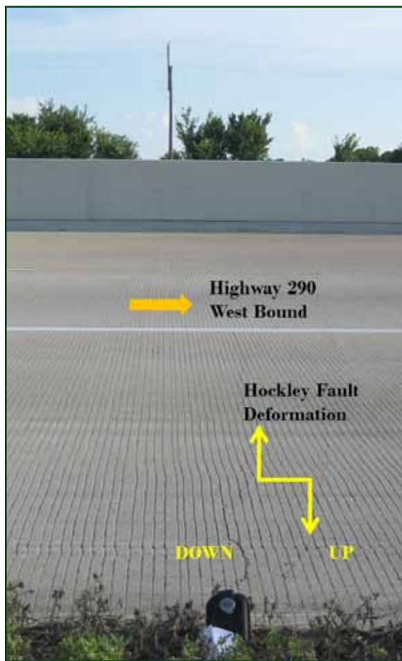
Figure 4. A recent picture (August 2010) showing revived cracks (main Hockley Fault) on the west bound of Highway 290. The fault deforms the newly built highway 290 and the feeder roads. The picture was taken facing south.
