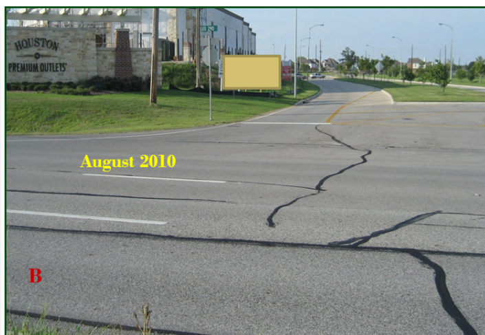
Figure 2. Recent pictures of Hockley Fault at Hwy. 290 Frontage and Fairfield Falls Way roads: A) taken in April 2010; B) taken in August 2010. Note the development of the tiny cracks in picture A into significant ones in picture B.
