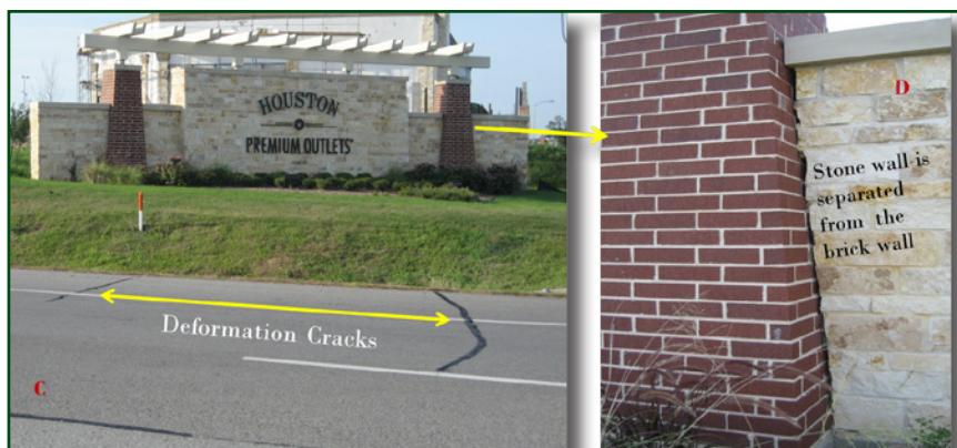
Figure 3. Pictures (C and D) of road and wall deformation to the immediate west of the Hockley Fault, respectively. The picture was taken in August 2010..
