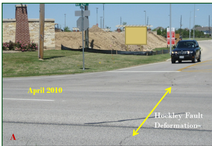
Figure 2. Recent pictures of Hockley Fault at Hwy. 290 Frontage and Fairfield Falls Way roads: A) taken in April 2010; B) taken in August 2010. Note the development of the tiny cracks in picture A into significant ones in picture B.
