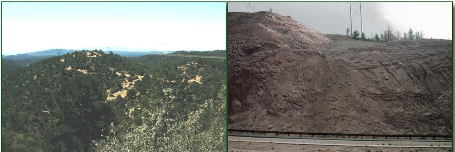
Figure 2. Views of rock cut area in weathered, fractured granites before and after excavation. The tower on the right is the replacement tower after the slope was re-engineered and reconstructed.
