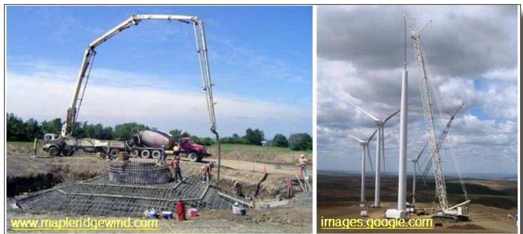
Figure 3. Turbine tower foundation construction (left) and tower-lifting crane (right).
